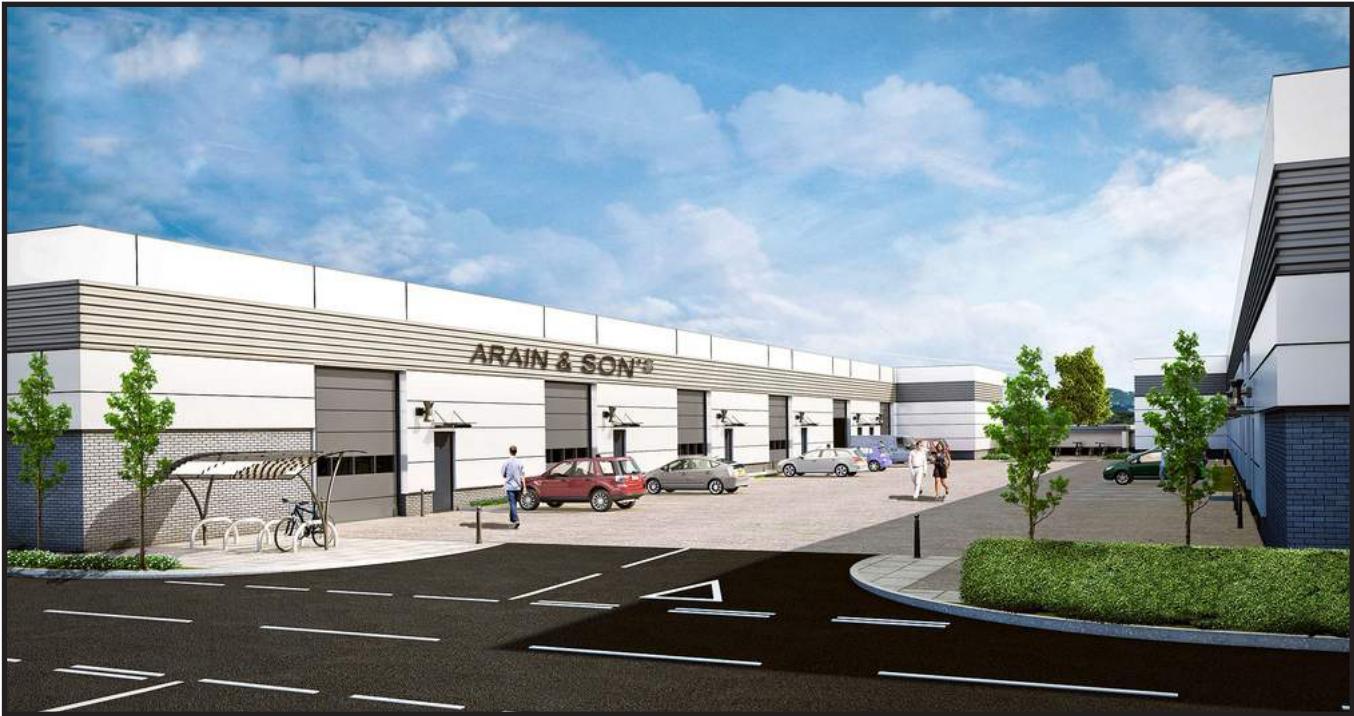
Under Construction Will be complete in Sep. 2018
